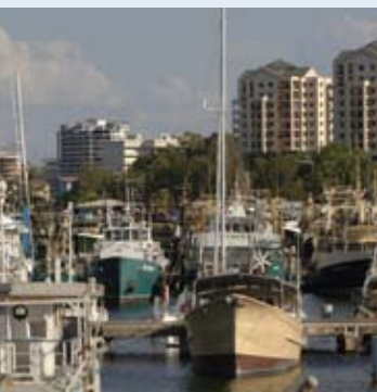
Darwin Wharf Precinct
